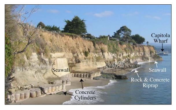
Figure 3: An unplanned assemblage of coastal armoring at Opal Cliffs in Capitola, California can have a visual impact on the beach user.
