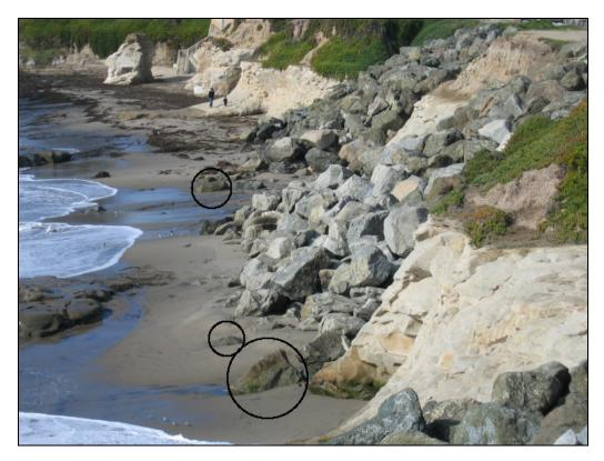
Figure 9: Riprap boulders commonly settle into deep sandy beaches or get buried, as seen here near the intersection of Westcliff Drive and David Street in Santa Cruz, California.
