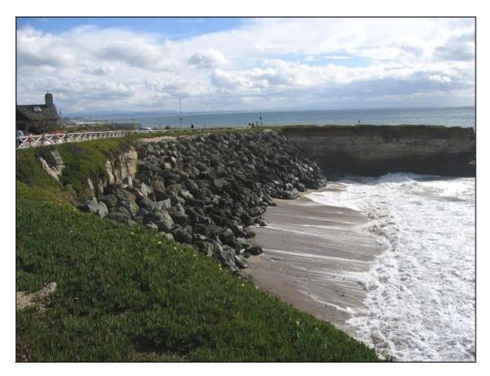
Figure 5: Riprap covering up significant amount of beach area in Santa Cruz, California, near the intersection of Westcliff Drive and San Jose Avenue.
