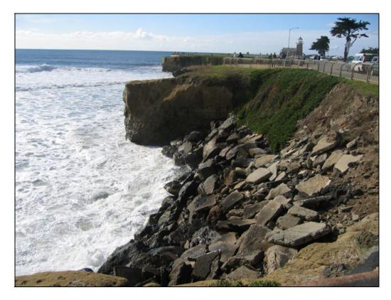
Figure 2: Concrete blocks used as riprap near Lighthouse Point in Santa Cruz, California.
