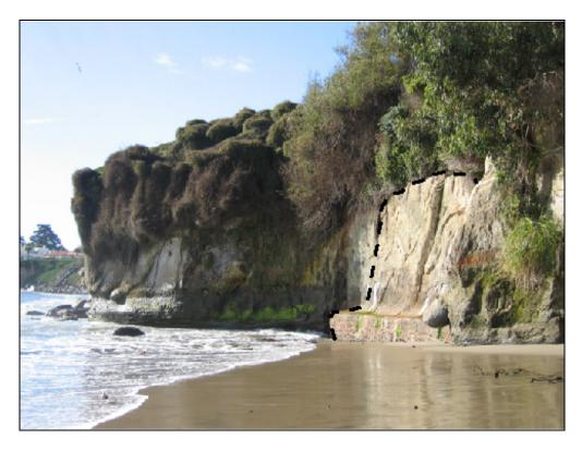
Figure 4: Photograph of cliff stabilization built to fill a seacave at Cowell's Beach in Santa Cruz. The 2004 gunite wall, outlined by the black dashed line, mimics the shape and color of the natural cliff.
