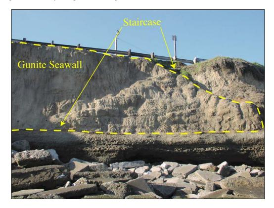
Figure 6: In this bluff stabilization project at Pleasure Point in Santa Cruz, the protective gunite (outlined with dotted line) was colored and textured to match the existing bluff materials, and access steps were built into the structure (Photograph by Gary Griggs).
