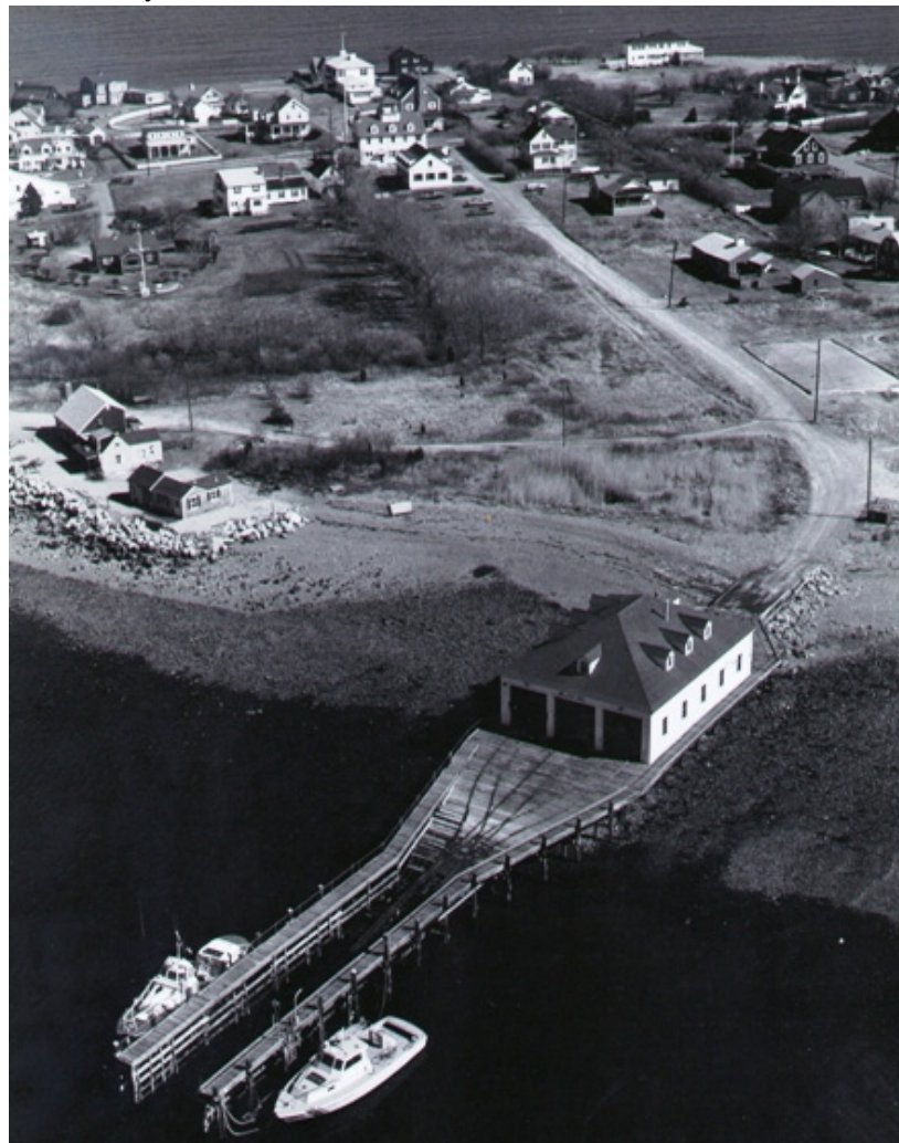
Significant structural changes to the campus buildings, including the removal of the marine railways, have contributed to the SBNMS facilities no longer being considered historic buildings under the Massachusetts Historical Commission. (Source: ONMS)
