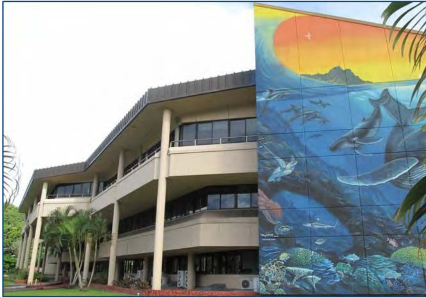
Photo 12: During the ASG-Convention Center renovations, AS DOC provided temporary sanctuary office space in the A.P. Lutali Executive Office Building, adorned with a Wyland mural commemorating the 2008 International Year of the Reef. Photo: Sarah Kinsfather.
