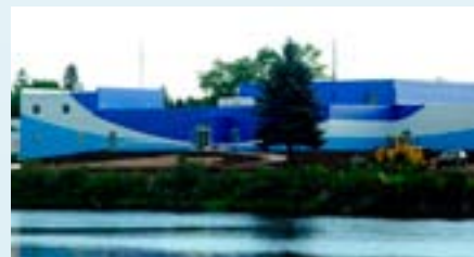
The Great Lakes Maritime Heritage Center in Alpena, MI, is a LEED® Gold building that features exhibits that explain building features that were designed to reduce energy consumption. Photo: ONMS
