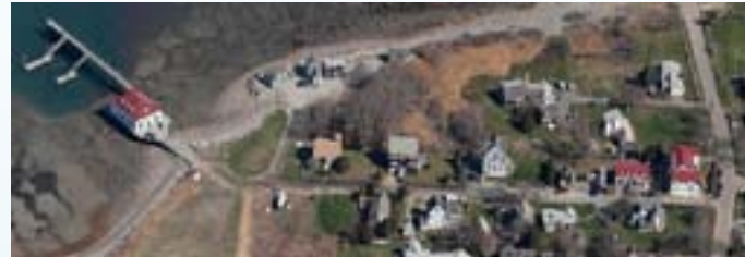
Aerial view of three Stellwagen Bank NMS buildings, denoted by red roofs, in Scituate, MA. The boathouse and pier (far left) will become a marine operations center. Photo: ONMS
